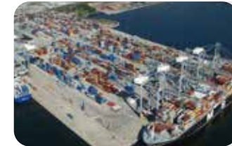
Coast And Port Structures
